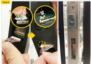
Plug the External Body Cable and the Door Position Sensor cable into Internal body circuit board. Place Internal body onto door stile. A clamp can be used to hold the External and Internal body on to the door, in preparation for the next step. Important: Plugs can only be installed one way. Do not use excessive force. Ensure the cables are not pinched and Internal body is aligned correctly with door mounting holes.
