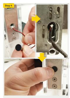
Feed Door Position Sensor wire through front mortice lock hole and exit out the internal side of door. Push Door Position Sensor firmly until it is flush with the lock faceplate.
