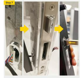
Feed the External body cable through lock cylinder hole. Place External body onto door stile, insert spindle through lock case and spindle hole in External body. A clamp can be used to hold the external body on to the door, in preparation for the next step. Important: Ensure the cable is not pinched and External body is aligned correctly with door mounting holes.
